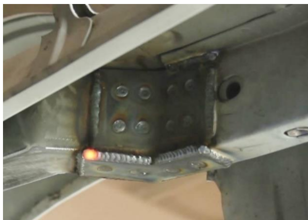
Figure 25 - Weld Bottom Frame Rail Doubler Plate
